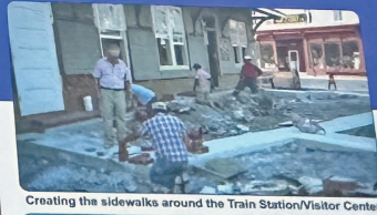
Creating the sidewalks around the Train Station/Visitor Center
