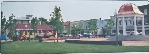
Final Stages of the Plaza
