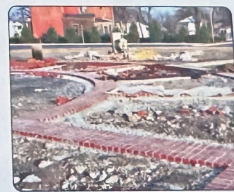
Brick work around the Gazebo
