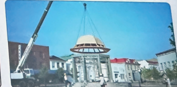
Hoisting the Dome atop the Gazebo
