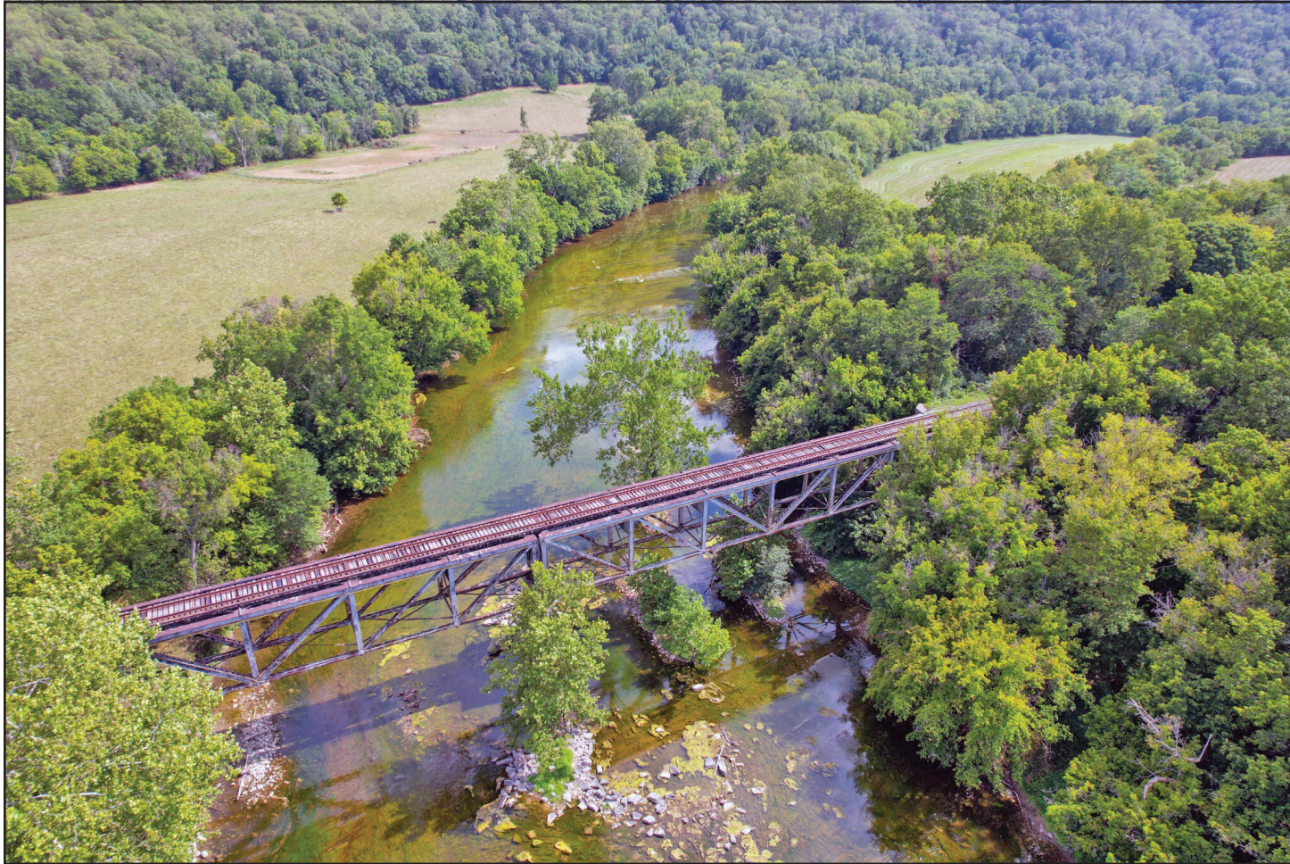
An aerial view of the bridge over the North Fork of the Shenandoah River. (Courtesy of Friends of the Shenandoah Rail Trail)
